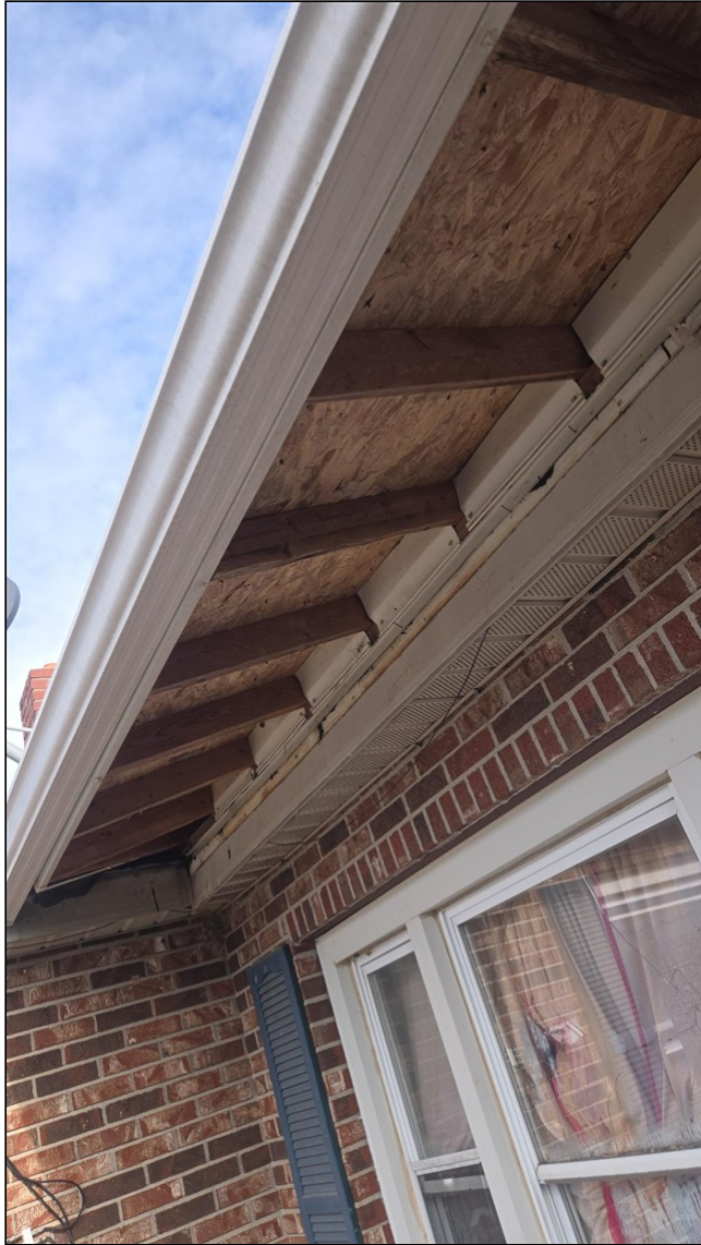
2.5 Item 1(Picture) There was missing soffit noticed.
