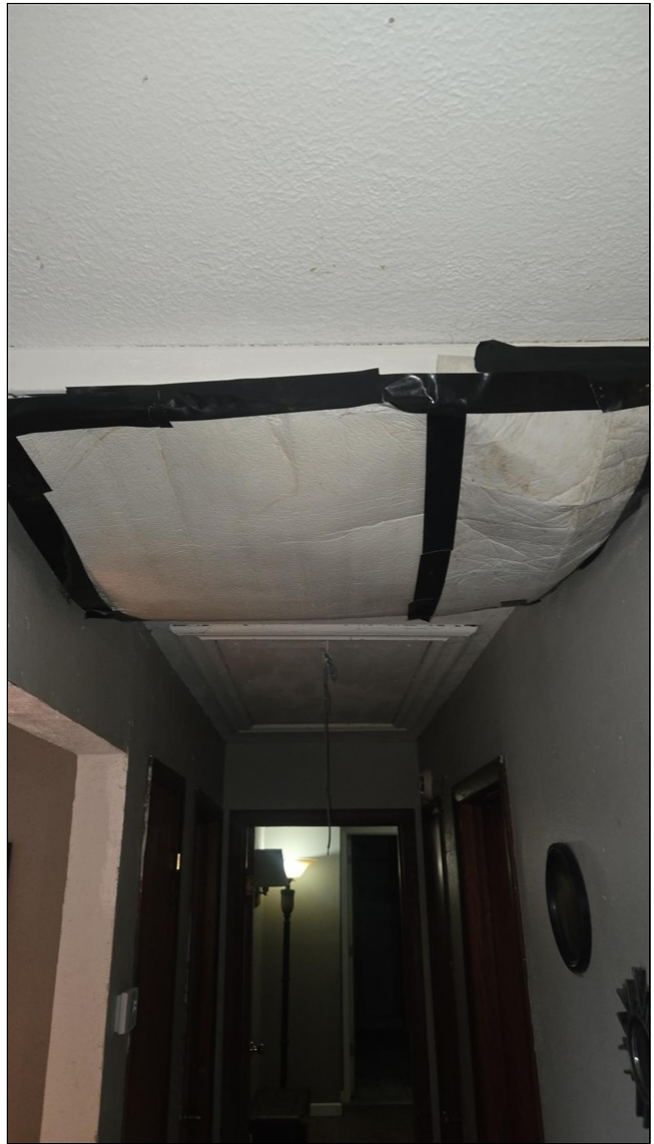
7.0 Item 2(Picture) The attic fan should be deleted and an attic access should be established here. InterNACHI recommends that attic fans are deleted, because overall they are less energy efficient than HVAC.
