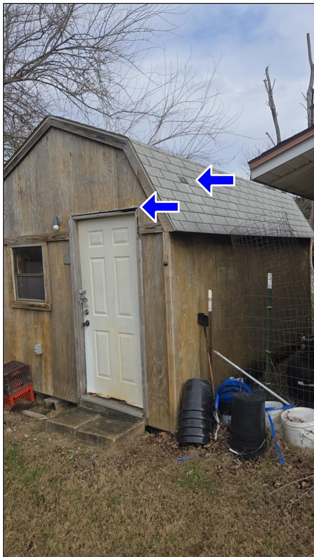
2.7 Item 1(Picture) There was exposed wood and metal. Exposed materials degrade faster than painted materials. A qualified contractor should repaint, stain, or seal any and all exposed materials. Painting of bare metal/wood is a minimum housing standard requirement.
