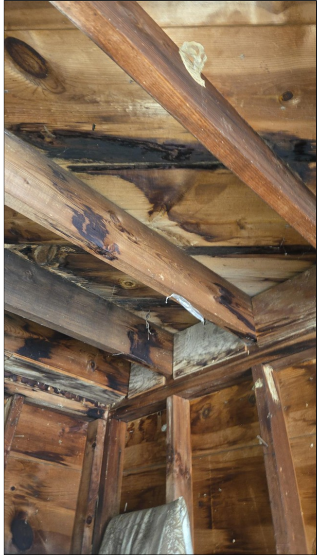
1.0 Item 2(Picture) There appeared to be active leaking and water damage in the area of the tree branches in the garage.
