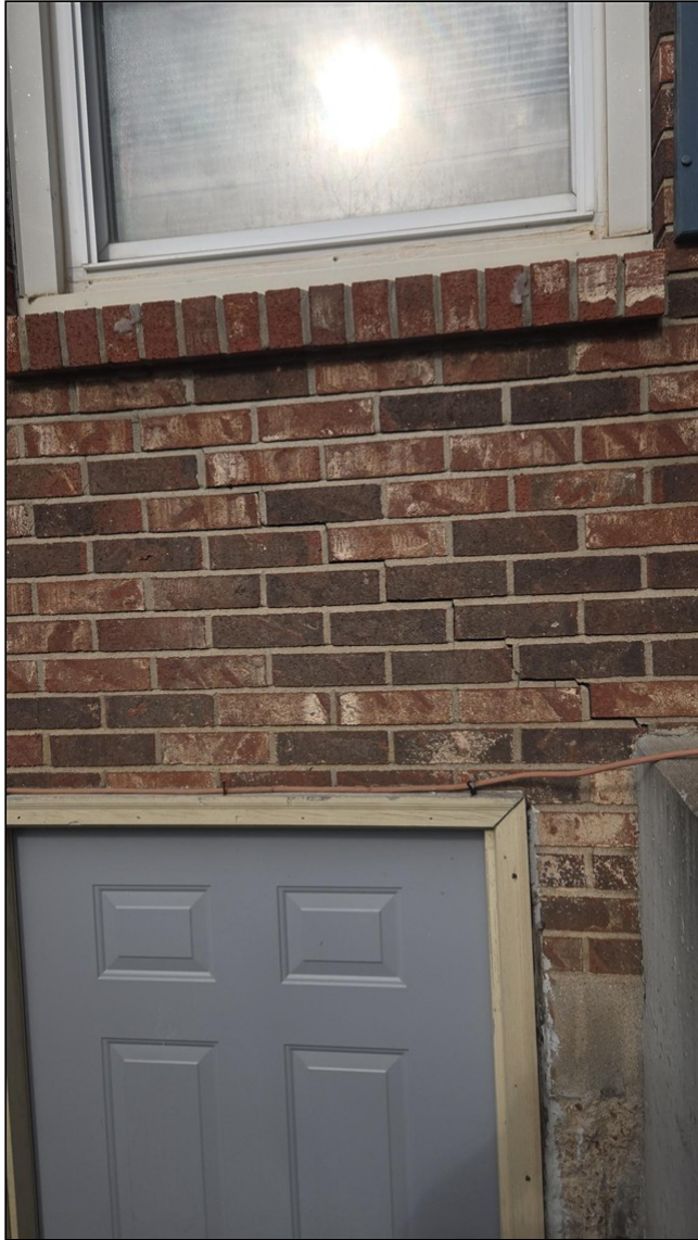
3.1 Item 3(Picture) The brick veneer required immediate repairs.
