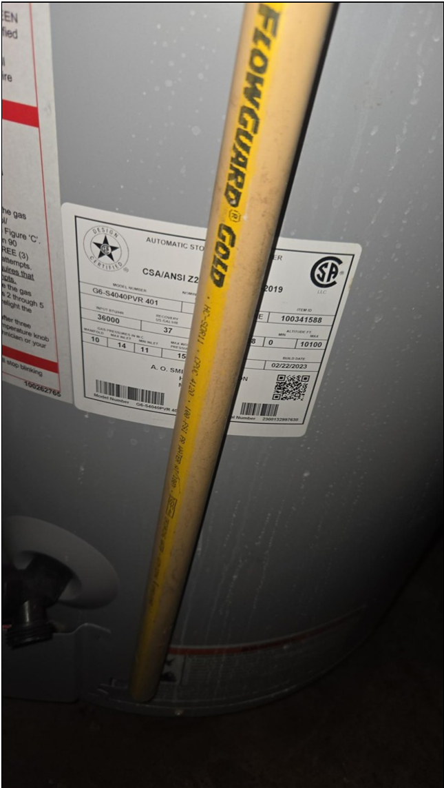
5.2 Item 2(Picture) 2008 AO Smith propane 40 gallon water heater inspected and operable at the time of the inspection. This unit is nearing the end of the useful life expectancy and may require repair or replacement during the period of ownership.
