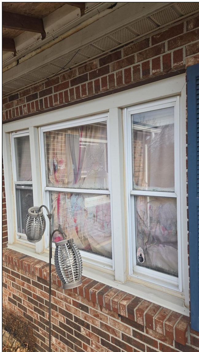
2.2 Item 1(Picture) Broken window - There was at least one broken window; any and all broken windows should be found and replaced by a qualified contractor. Minimum housing standards require all windows to be whole; exterior windows should open, close, latch, and lock. A qualified contractor should find and fix any and all broken or damaged windows.
