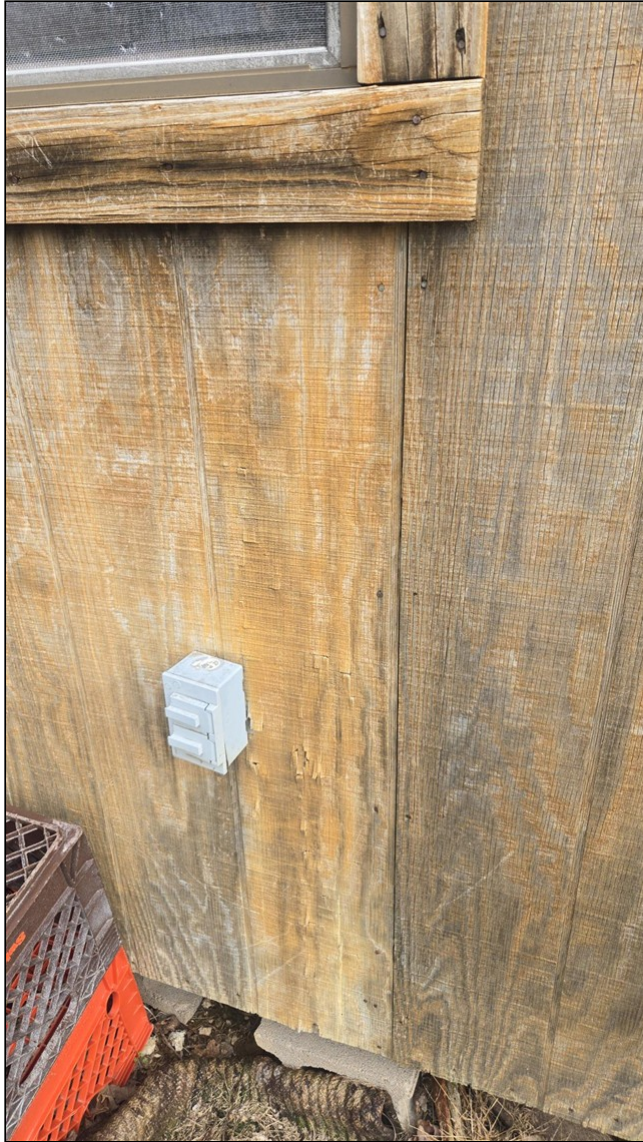
2.7 Item 3(Picture) Bare wood. Not GFCI protected. Outbuilding electrical systems do not meet National Electrical code guidelines. A licensed electrical contractor should bring all of the buildings and the pool area up to modern standards.
