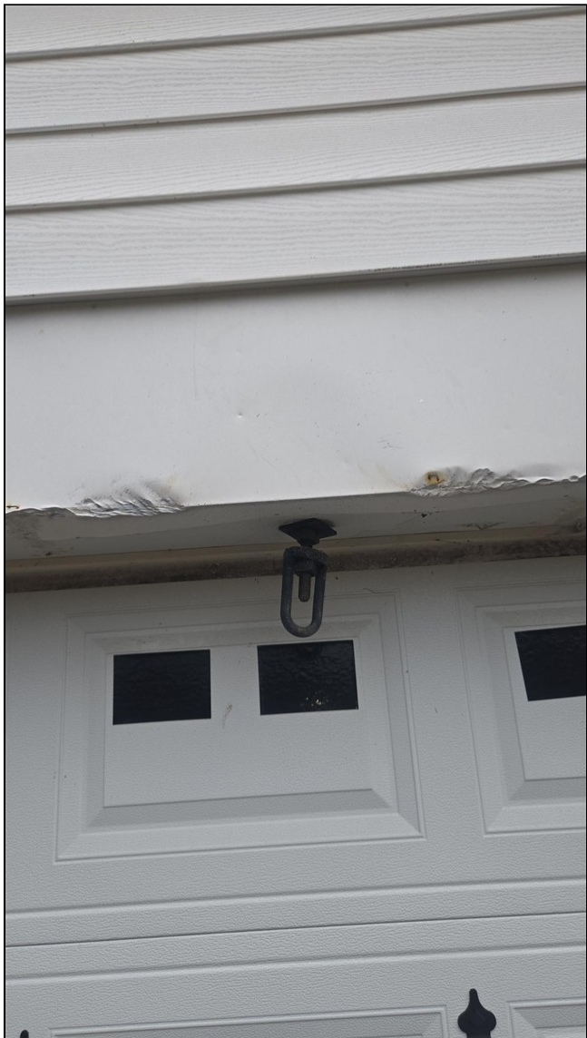
2.7 Item 9(Picture) Damaged outbuilding fascia.
