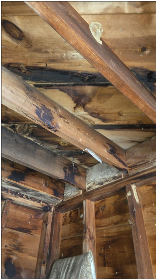
1.0 Item 2(Picture) There appeared to be active leaking and water damage in the area of the tree branches in the garage.
