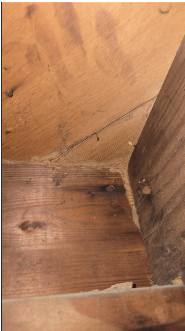
3.3 Item 4(Picture) Floor joist termite damage noticed. There was noticeable deflection in the floors in some areas and I expect that there are some floor joists that require repairs. Evidence of termites and some termite damage was found. Some termite damage may be hidden. We recommend termite treatment. Any and all termite damaged wood should be repaired or replaced. A qualified contractor should repair or replace any and all damaged, cracked, or buckled floor joists. The floor joists should be sistered with a continuous board that is the same size as width as the existing floor joist and the same length as the existing floor joist. The sistered floor joist should be bearing on the sill plate on one side and bearing on the beam on the otherside. The sistered floor joist should be #6 screwed or 6d nailed to the old floor joist on an eschelon pattern with 6" offset between the fasteners. The fasteners should alternate between top and bottom of the floor joist. The fasteners should not be located less than 2" from the outside edge of the board. The sistered board should be installed crown facing up.
