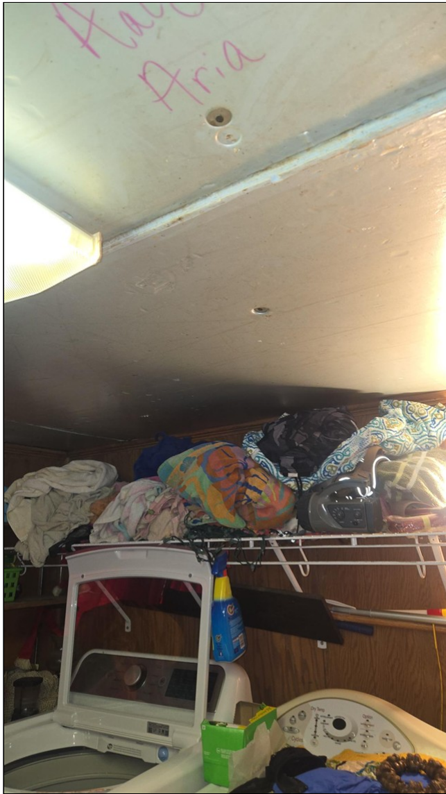
7.0 Item 1(Picture) There was not a finished ceiling in the laundry room. This ceiling should be removed and the wood rafters should be inspected in this area prior to finishing this ceiling. There may be hidden water damage in this area.
