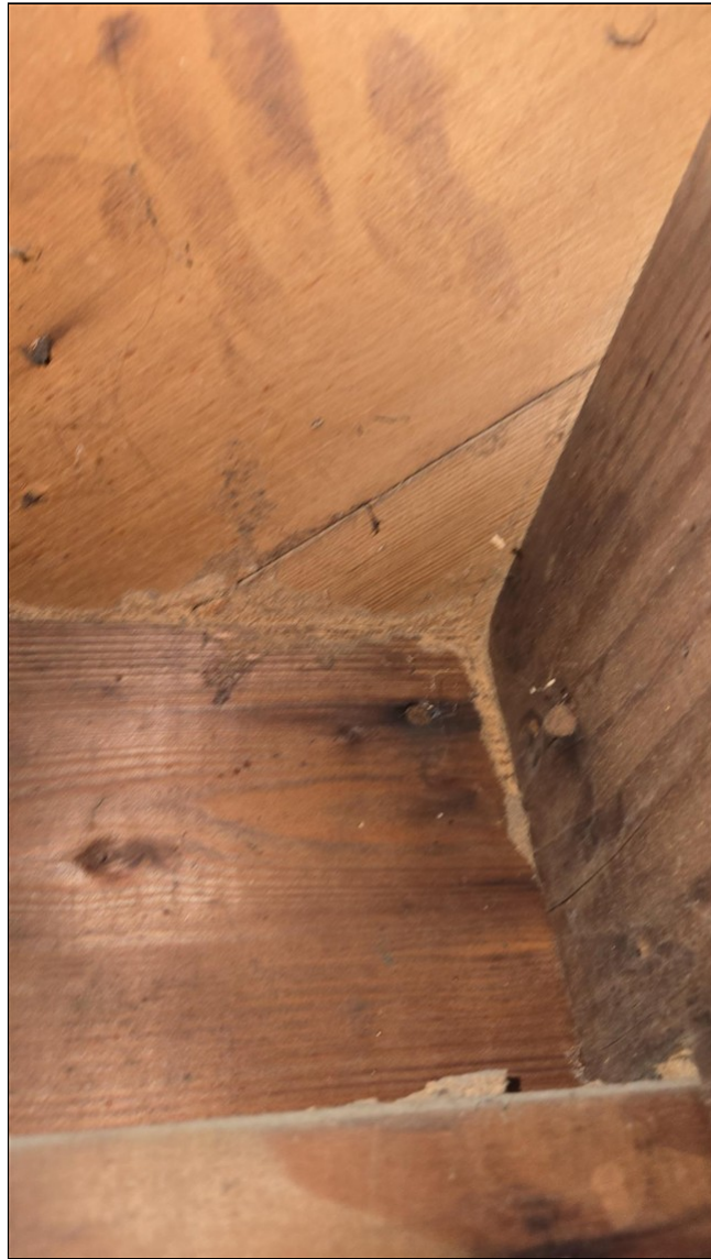
3.3 Item 4(Picture) Floor joist termite damage noticed. There was noticeable deflection in the floors in some areas and I expect that there are some floor joists that require repairs. Evidence of termites and some termite damage was found. Some termite damage may be hidden. We recommend termite treatment. Any and all termite damaged wood should be repaired or replaced. A qualified contractor should repair or replace any and all damaged, cracked, or buckled floor joists. The floor joists should be sistered with a continuous board that is the same size as width as the existing floor joist and the same length as the existing floor joist. The sistered floor joist should be bearing on the sill plate on one side and bearing on the beam on the otherside. The sistered floor joist should be #6 screwed or 6d nailed to the old floor joist on an eschelon pattern with 6" offset between the fasteners. The fasteners should alternate between top and bottom of the floor joist. The fasteners should not be located less than 2" from the outside edge of the board. The sistered board should be installed crown facing up.
