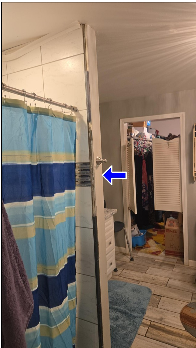
7.1 Item 5(Picture) The master bathroom shower wall looked like it may have some major rot and water damage behind the wall. This wall should be torn down to the studs and inspected.
