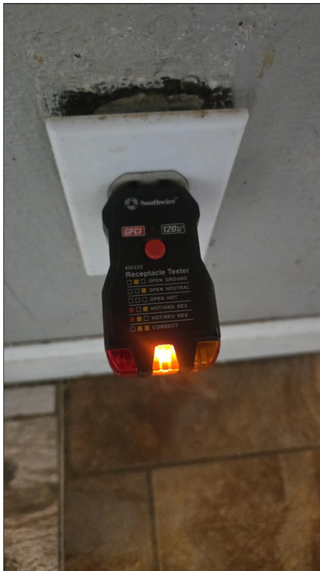
6.3 Item 4(Picture) Ungrounded outlets throughout the house. A qualified electrical contractor should find and fix any and all National Electrical Code deficiencies.
