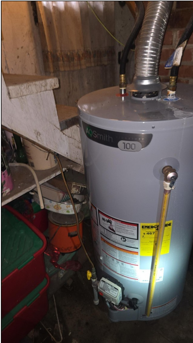
5.2 Item 1(Picture) 2008 AO Smith propane 40 gallon water heater inspected and operable at the time of the inspection. This unit is nearing the end of the useful life expectancy and may require repair or replacement during the period of ownership.
