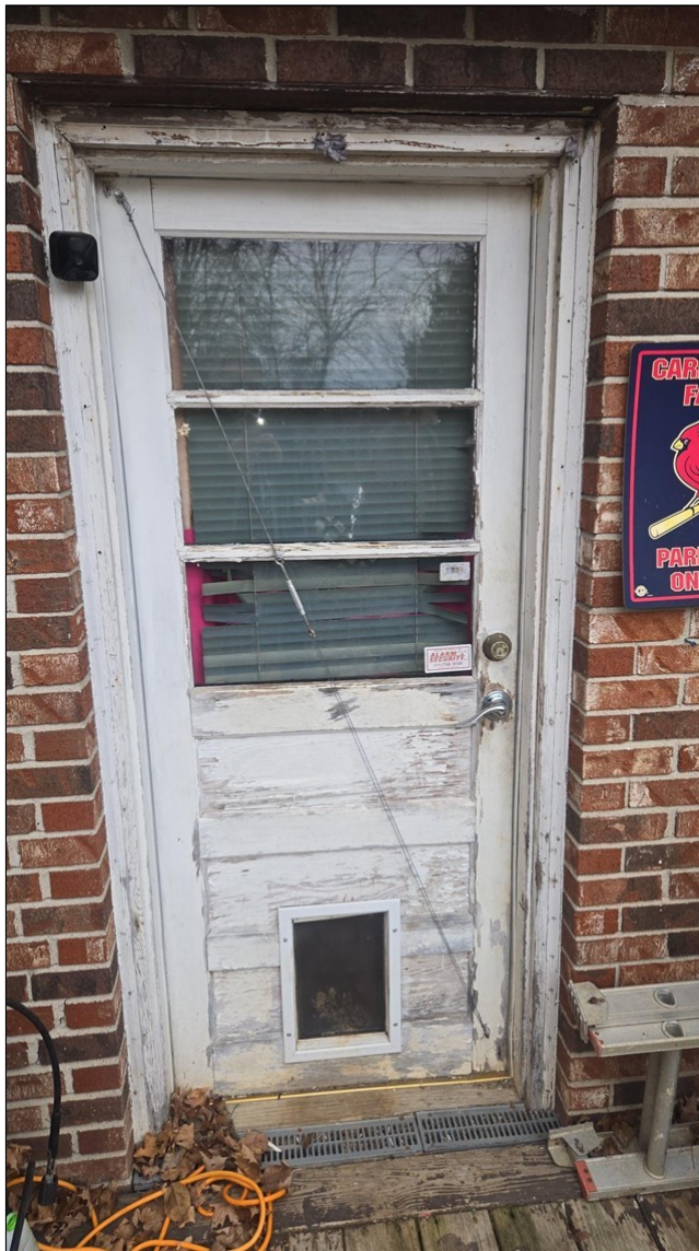
2.1 Item 4(Picture) There was bare wood and rotted wood noticed. There was exposed wood and metal. Exposed materials degrade faster than painted materials. A qualified contractor should repaint, stain, or seal any and all exposed materials. Painting of bare metal/wood is a minimum housing standard requirement.
