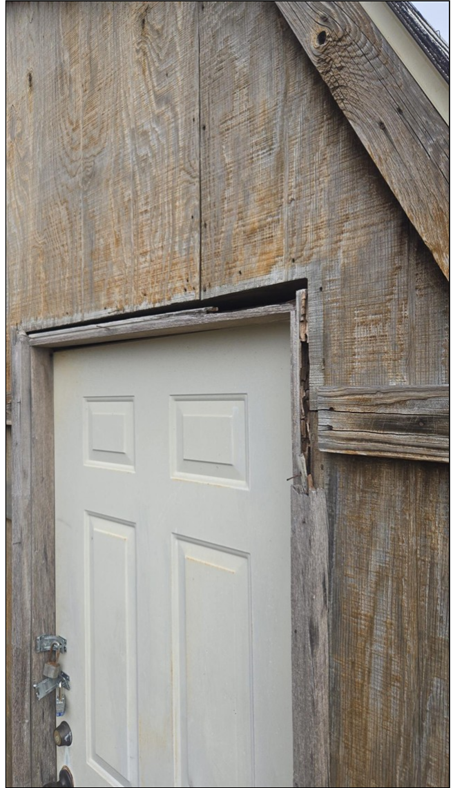
2.7 Item 10(Picture) Rotted wood outbuilding.
