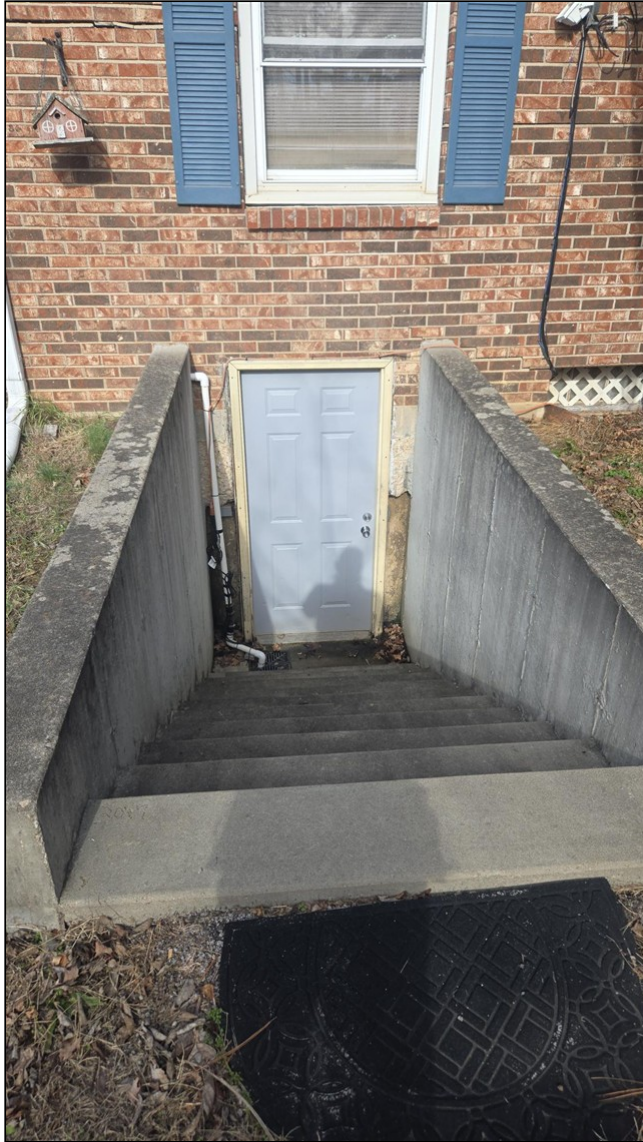
2.3 Item 1(Picture) Missing handrail. Handrails should be designed to handle 300# of force applied in any direction. Handrails should also be graspable by wrapping a hand completely around the handrail to help prevent slips, trips, and falls. Every stairwell with 4 risers or more should have a handrail. A qualified contractor should repair the handrails that don't meet those requirements.
