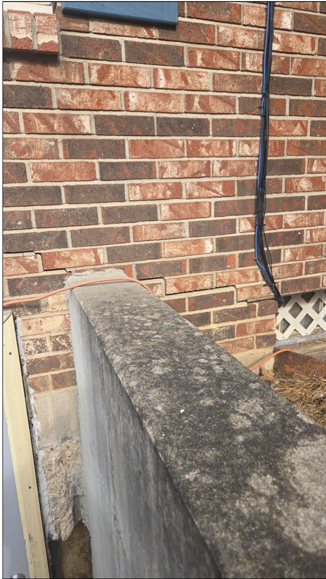
3.1 Item 4(Picture) The brick veneer required immediate repairs.
