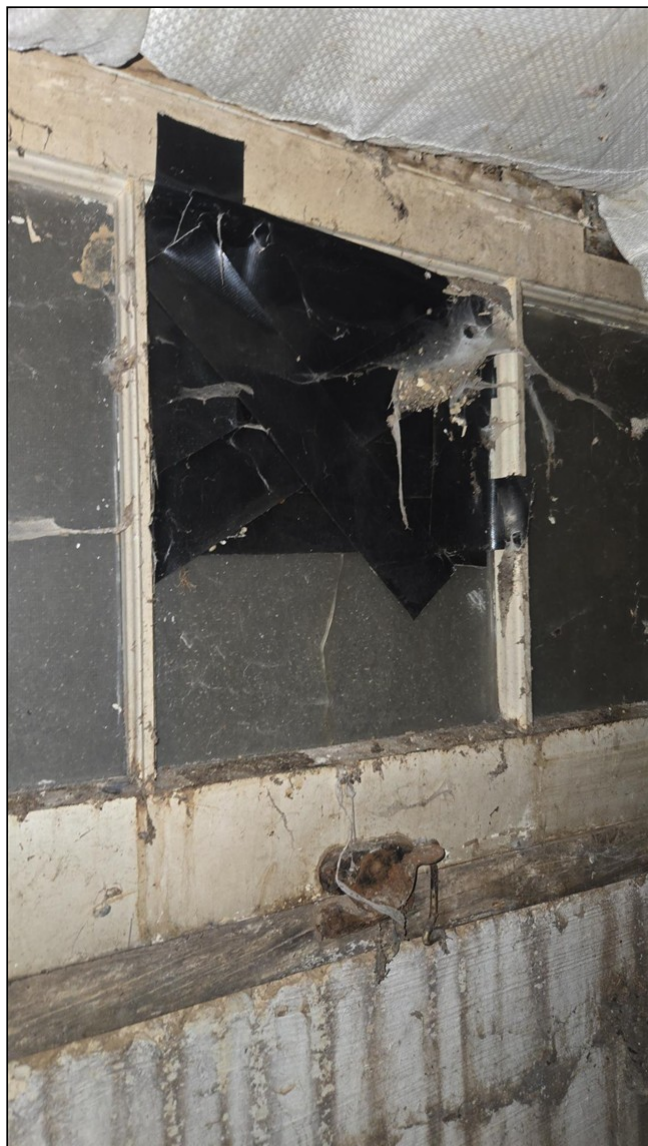
7.6 Item 3(Picture) Broken basement crawlspace entrance.
