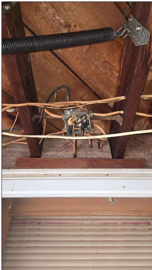
6.3 Item 1(Picture) Open and overloaded splice boxes - A qualified electrical contractor should find and fix any and all National Electrical Code deficiencies.
