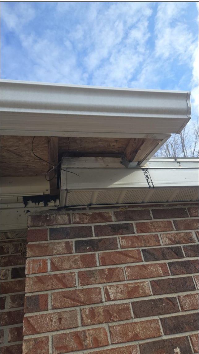
1.1 Item 2(Picture) The flashing on the roof between the flat roof and the house was missing and did not look appropriate. This is an unusual situation and it should be repaired by a qualified roofer. This situation may cause leaks and there may be hidden water damage in this area.
