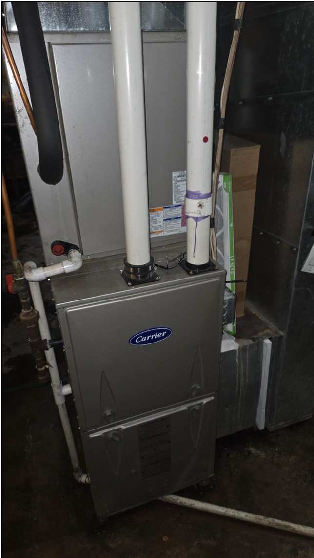
4.0 Item 1(Picture) 2016 Carrier gas furnace inspected and operable at the time of the inspection.
