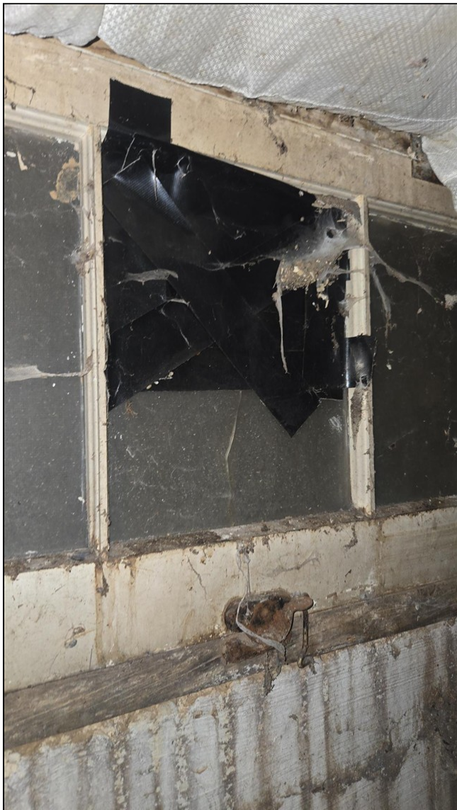
7.6 Item 3(Picture) Broken basement crawlspace entrance.
