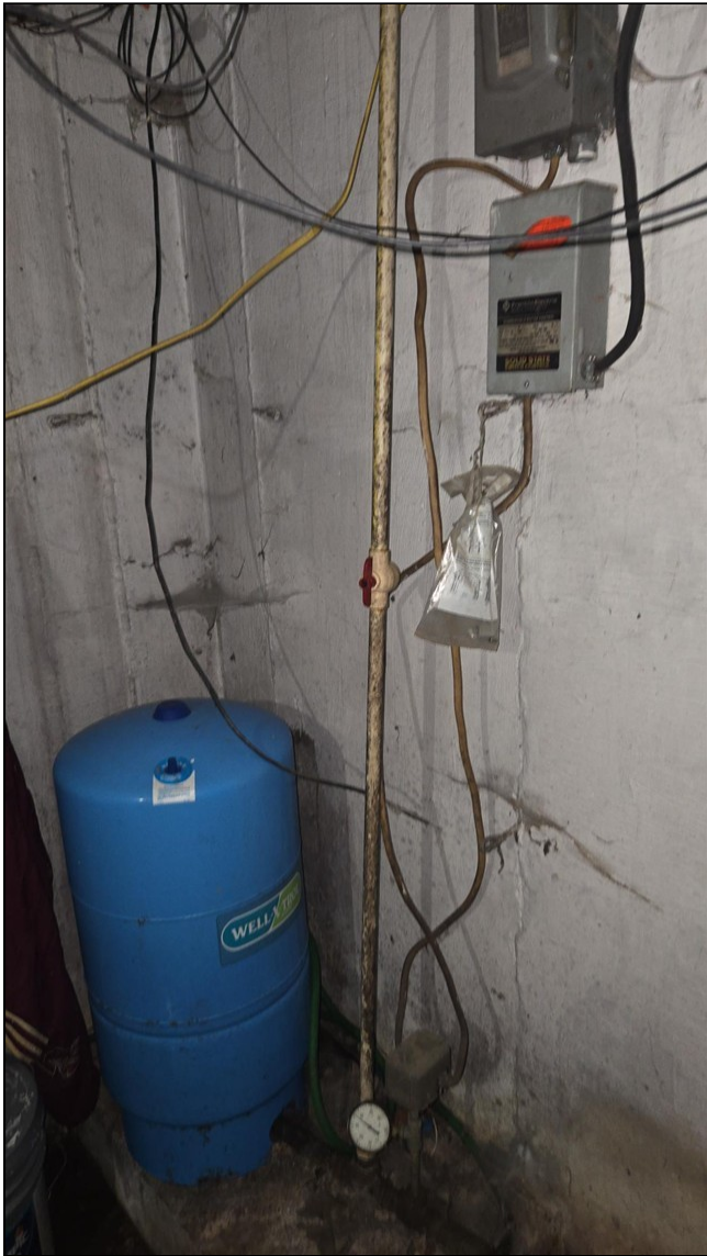
5.1 Item 3(Picture) This pressure tanks should be drained and de-scaled.
