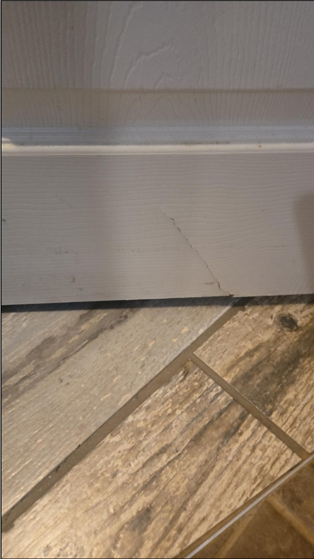
7.5 Item 7(Picture) Cracked door.
