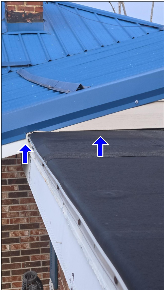
1.1 Item 1(Picture) The flashing on the roof between the flat roof and the house was missing and did not look appropriate. This is an unusual situation and it should be repaired by a qualified roofer. This situation may cause leaks and there may be hidden water damage in this area.
