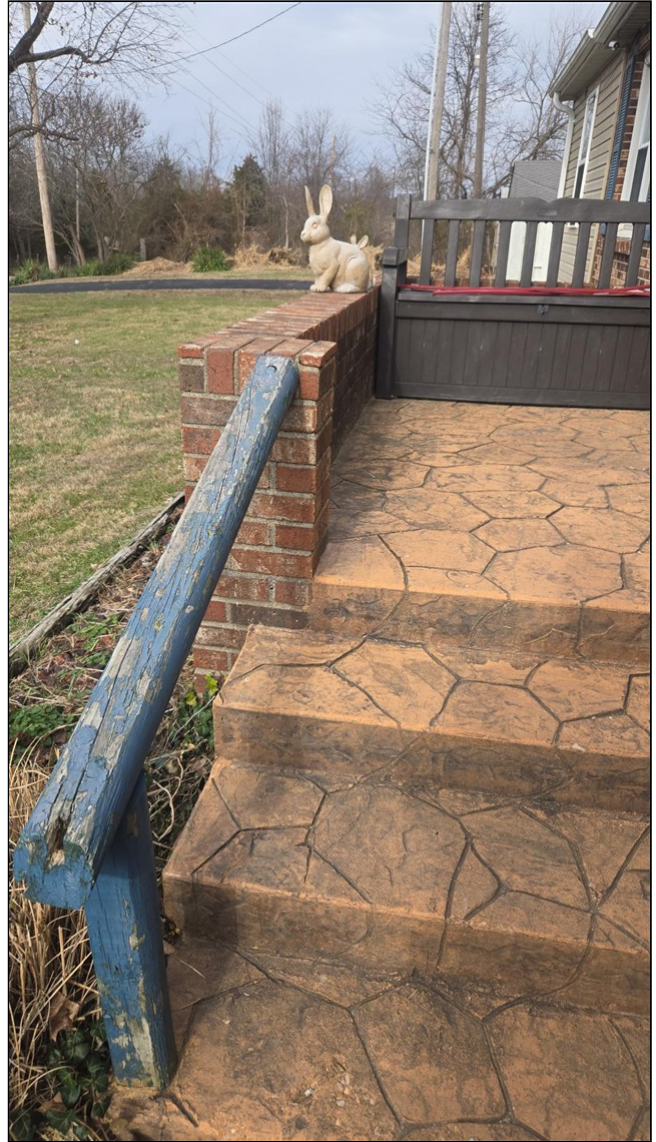
2.3 Item 2(Picture) There was bare wood and rotted wood noticed. There was exposed wood and metal. Exposed materials degrade faster than painted materials. A qualified contractor should repaint, stain, or seal any and all exposed materials. Painting of bare metal/wood is a minimum housing standard requirement.
