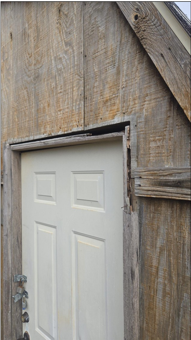
2.7 Item 10(Picture) Rotted wood outbuilding.
