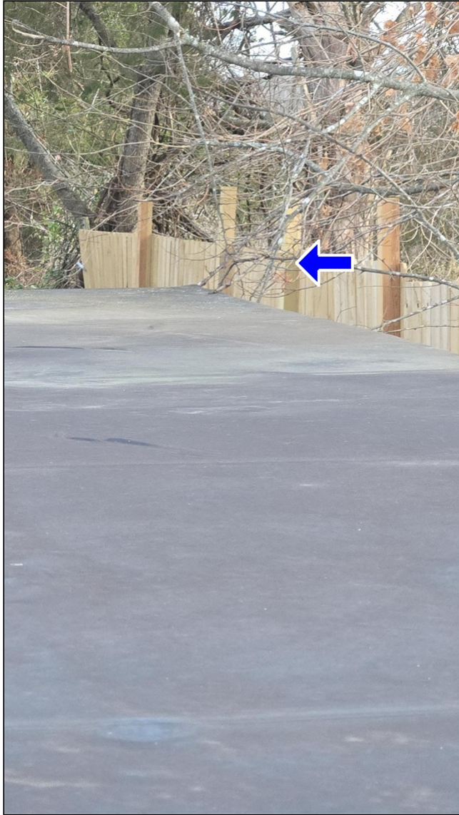
1.0 Item 1(Picture) Tree branches should be cut back 6' outside of the perimeter of the home plumb to the sky. Tree branches that are closer to the home than that may cause sudden damage and leaking.
