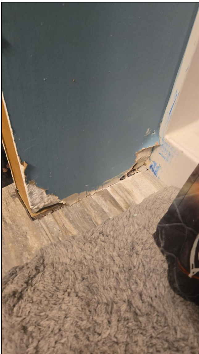
7.1 Item 3(Picture) There were drywall repairs required.
