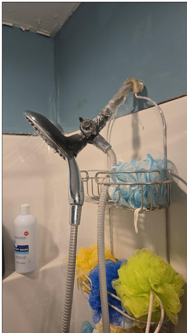
5.1 Item 2(Picture) This shower head leaked and required repairs.
