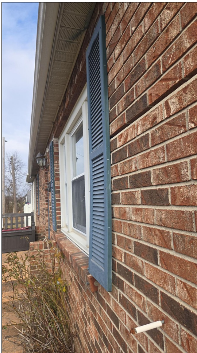
2.2 Item 2(Picture) Loose shutter - There was at least one loose shutter.
