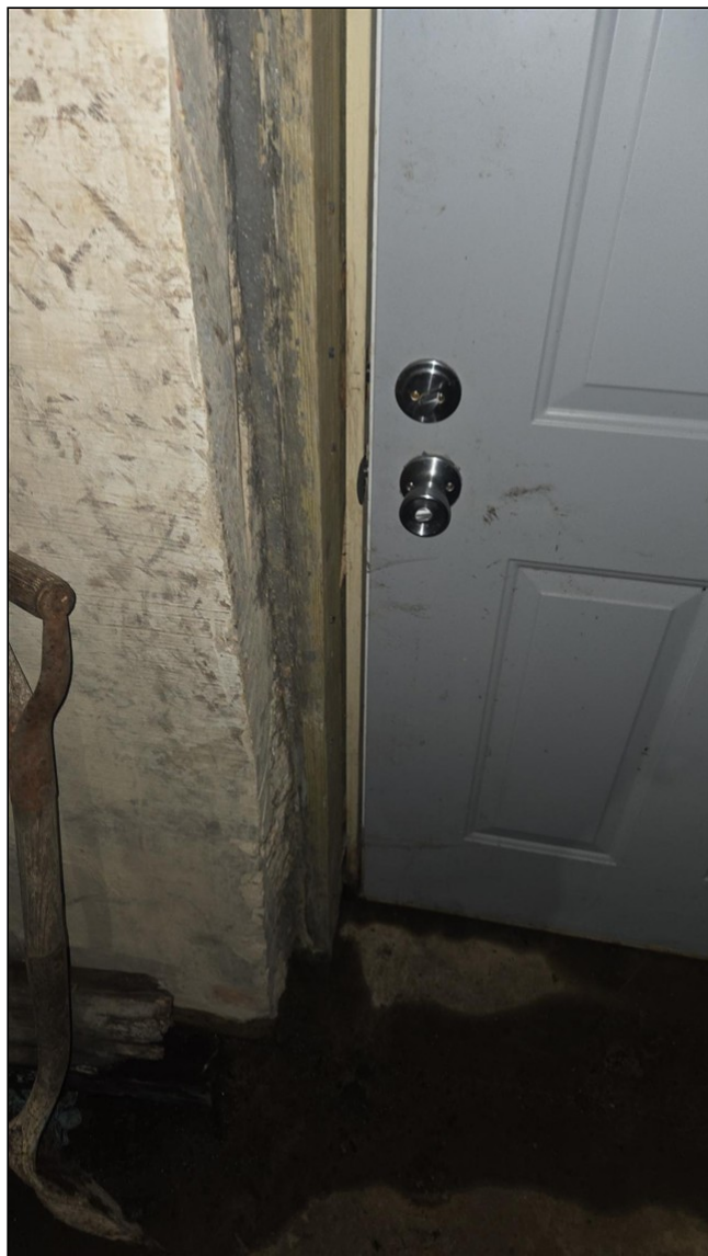
2.1 Item 3(Picture) Bolt doesn't lock on basement door. The basement door required repair.
