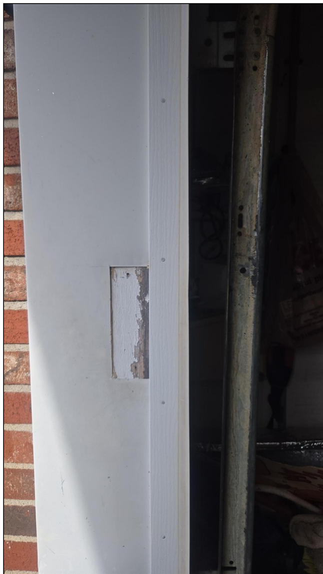
8.3 Item 1(Picture) The garage door fascia required repairs.
