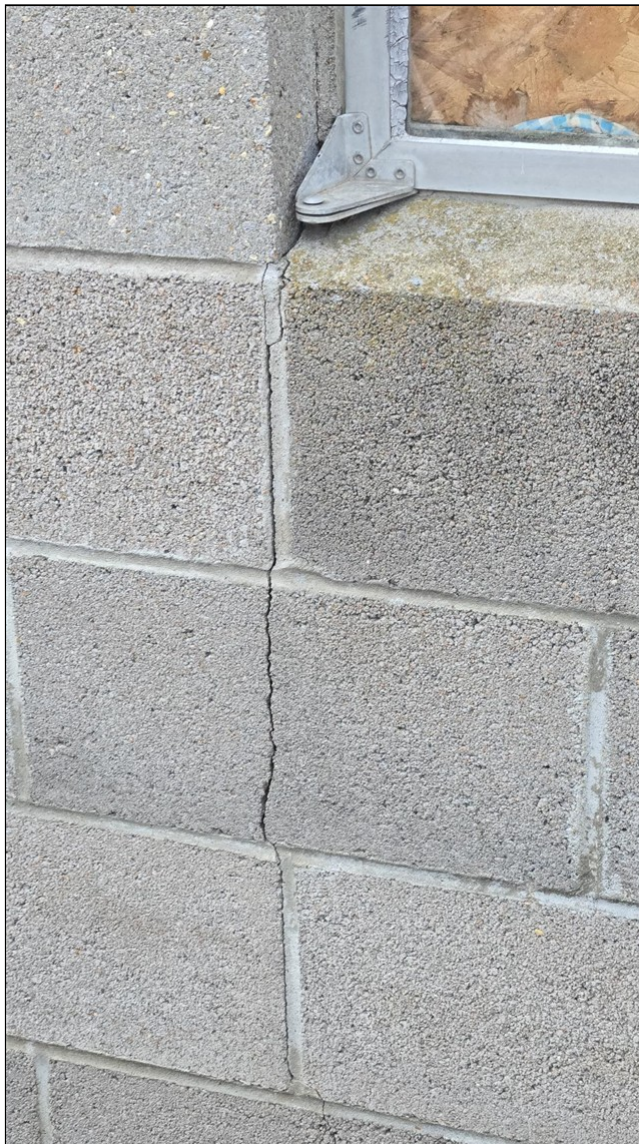
2.7 Item 8(Picture) Masonry repairs required to outbuilding.
