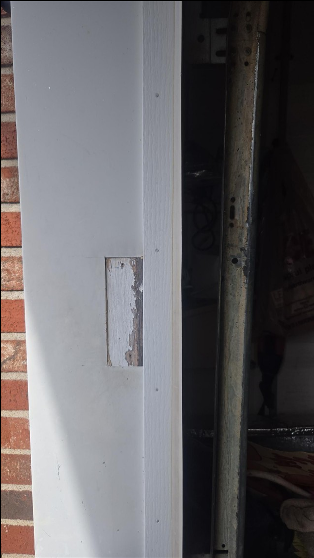
8.3 Item 1(Picture) The garage door fascia required repairs.
