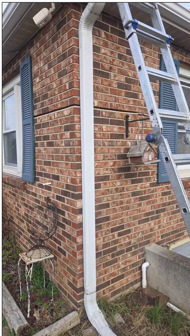
3.1 Item 1(Picture) The brick veneer required immediate repairs.
