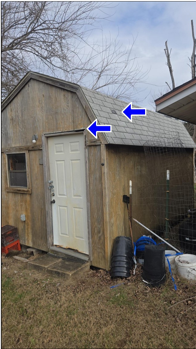
2.7 Item 1(Picture) There was exposed wood and metal. Exposed materials degrade faster than painted materials. A qualified contractor should repaint, stain, or seal any and all exposed materials. Painting of bare metal/wood is a minimum housing standard requirement.
