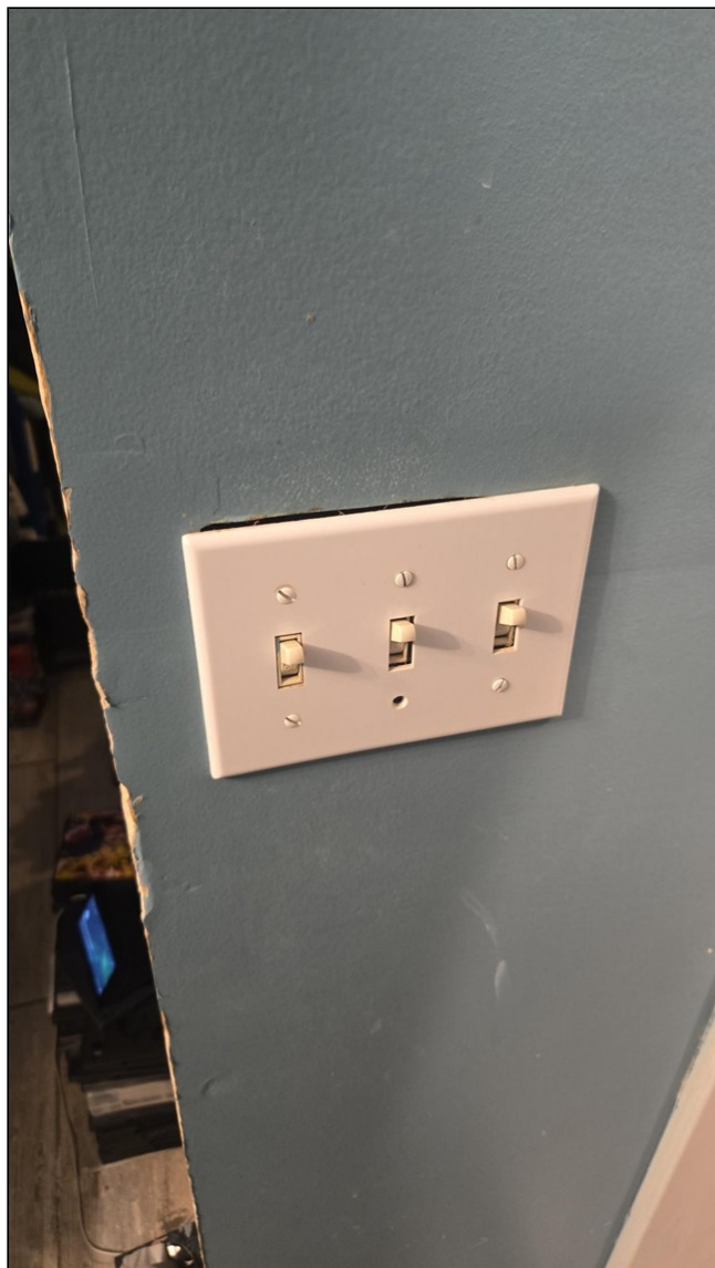
6.3 Item 5(Picture) A qualified electrical contractor should find and fix any and all National Electrical Code deficiencies. Missing screws, cracked covers, covers loose or protruding from the wall.
