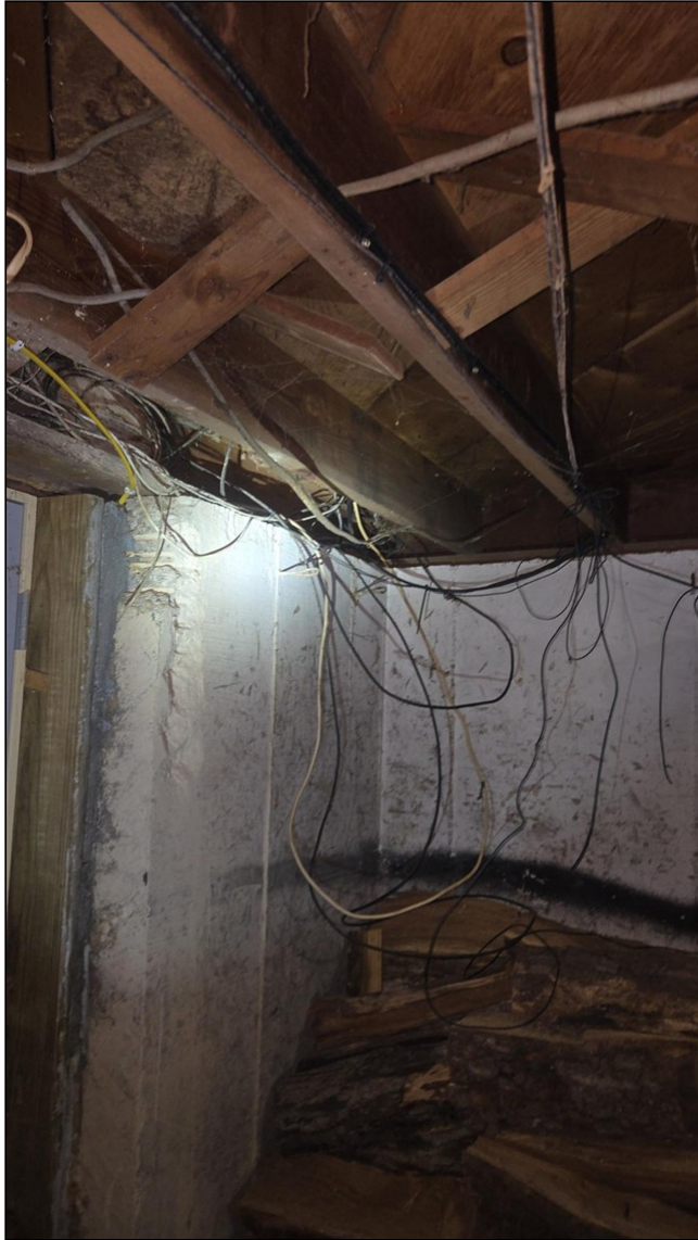
6.3 Item 7(Picture) A qualified electrical contractor should find and fix any and all National Electrical Code deficiencies. Loose wires
