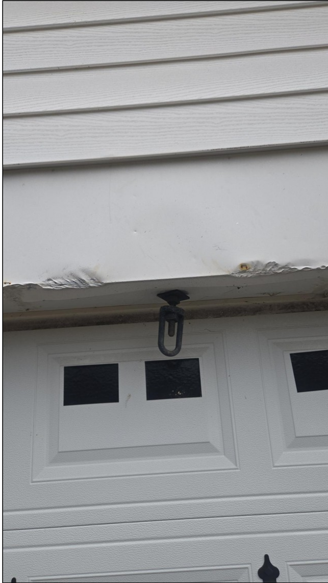
2.7 Item 9(Picture) Damaged outbuilding fascia.
