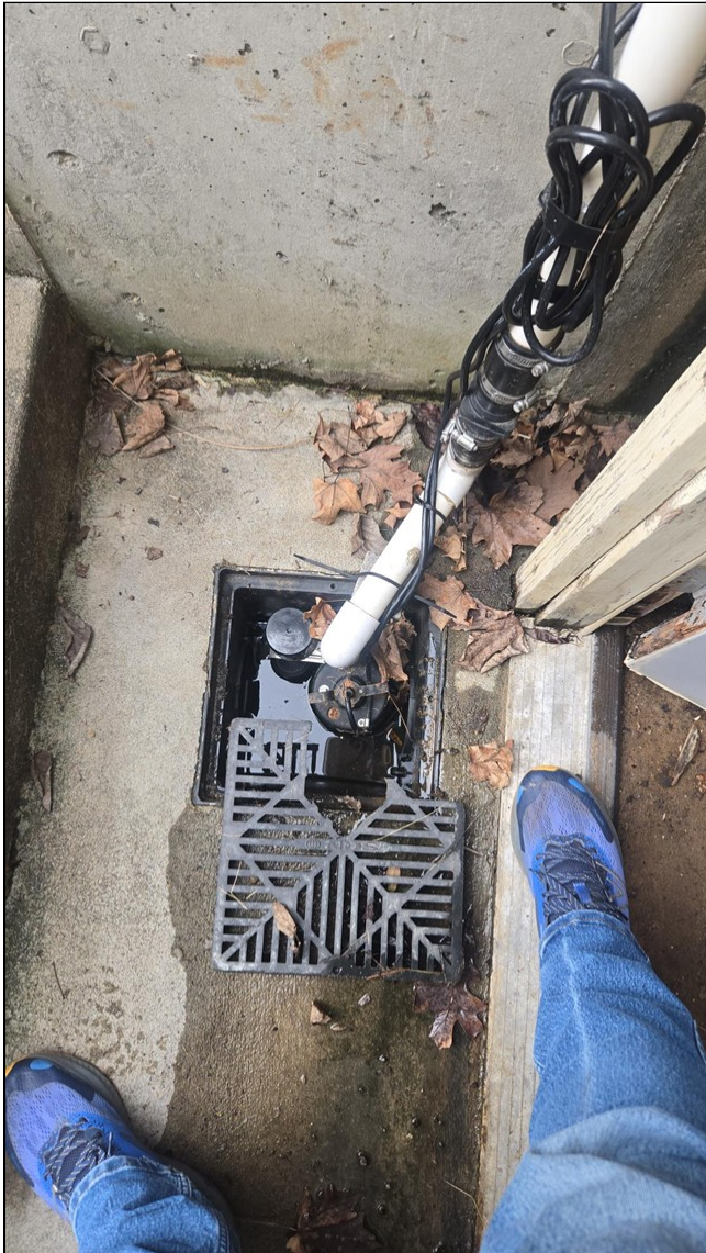
5.5 Item 1(Picture) The sump at the bottom of the basement stairwell was operable at the time of the inspection.
