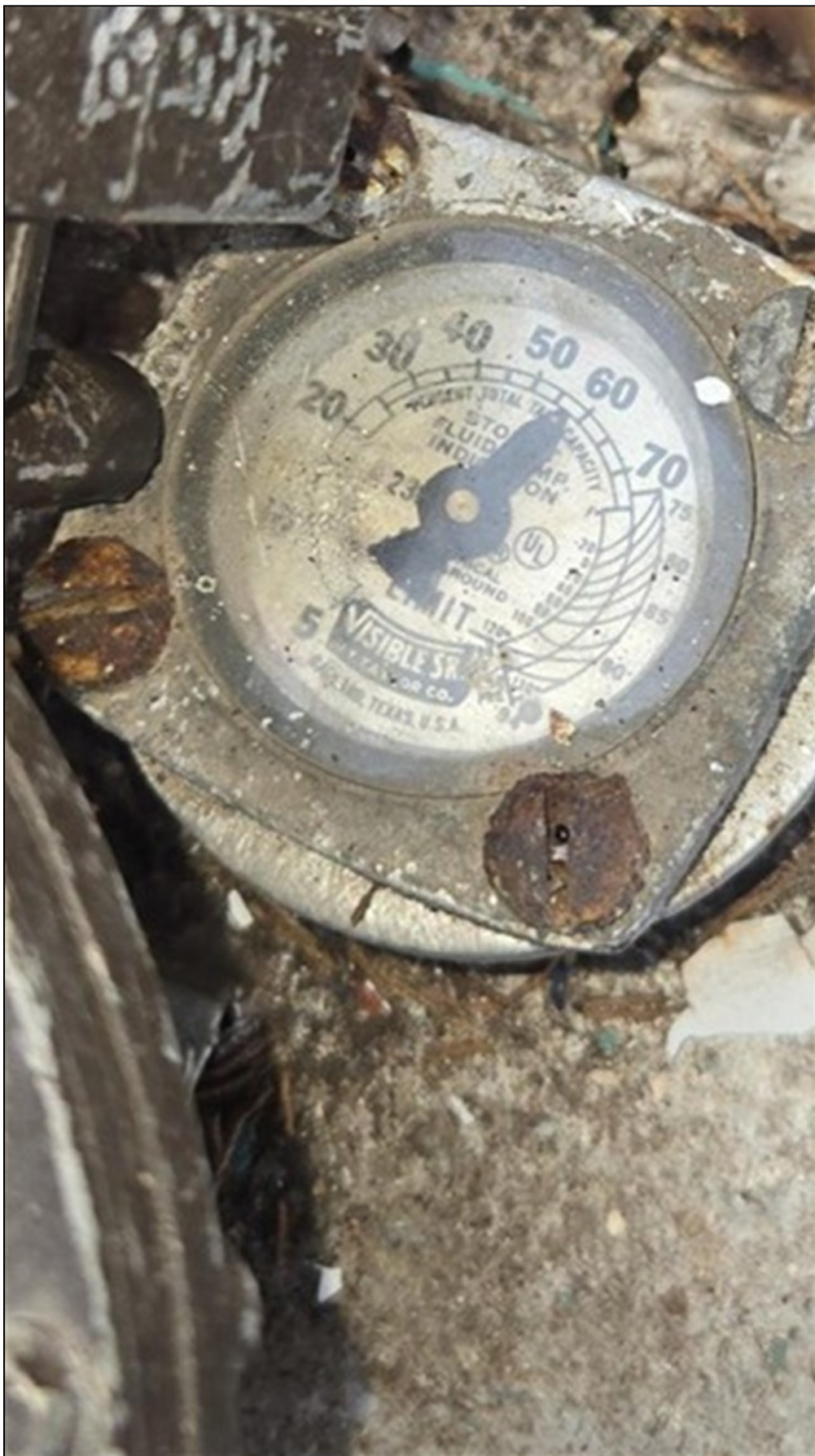
5.4 Item 2(Picture) The tank pop off valves should be serviced by the tank provider. The main gas shut-off valve is located at the propane tank. The tank was 57% full at the time of the inspection.
