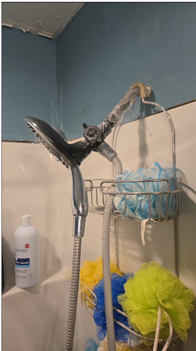
5.1 Item 2(Picture) This shower head leaked and required repairs.
