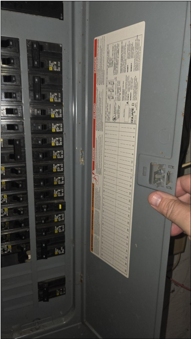
6.1 Item 4(Picture) Breakers not labeled. A qualified electrical contractor should find and fix any and all National Electrical Code deficiencies.
