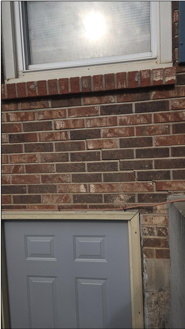
3.1 Item 3(Picture) The brick veneer required immediate repairs.
