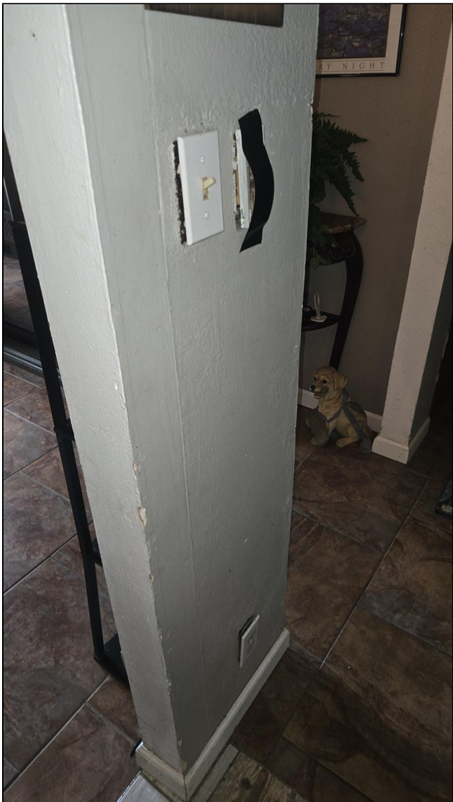
6.3 Item 3(Picture) Outlets and switches should all be replaced and properly installed. A qualified electrical contractor should find and fix any and all National Electrical Code deficiencies.
